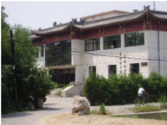
Photograph 2. The National Laboratory of Protein Engineering and Plant Genetic Engineering
